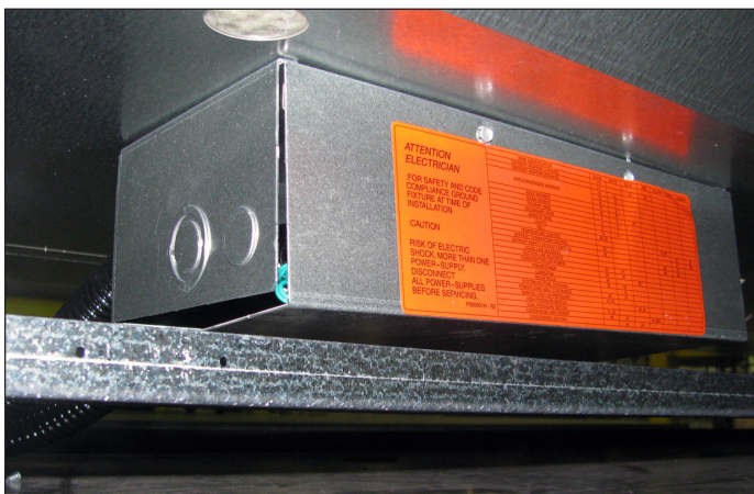
Fig. 12 Junction box beneath case
