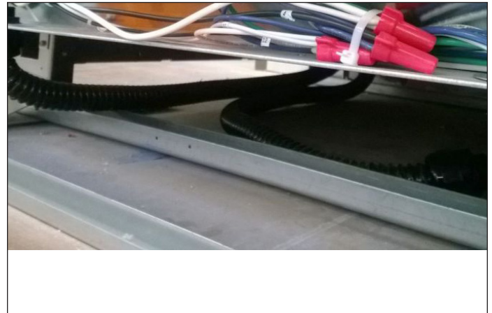
Fig. 13 Raceway wiring
