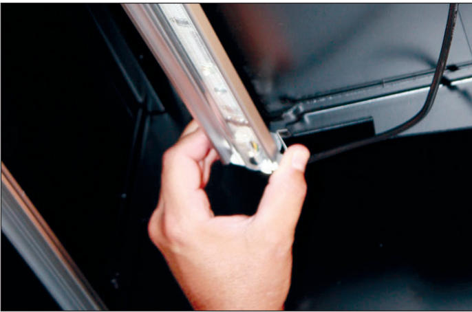
Fig. 19 Remove the old LED luminaire.
